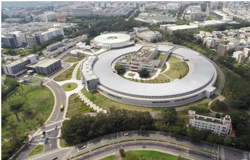
Figure 1: An aerial photograph of the NSRRC. This photograph shows the recently completed TPS and the 21-year-old Taiwan Light Source (TLS). The proposal of the TPS project was prepared in 2004. The civil construction of the TPS began in February 2010, and was completed in December 2013. The assembly of main accelerator parts was completed in 2014. The TPS project came to realization after ten years of efforts.
